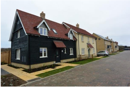
Hill Farm, Foxton (new council homes) Finalist – Building Excellence Awards 2018 Best social or affordable new housing development
